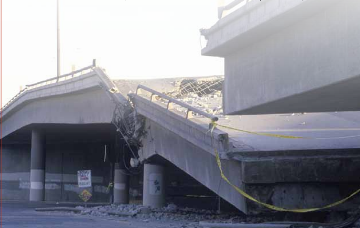
1994, highway in the Northridge residential area at the epicenter of the earthquake
