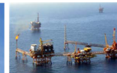
Oil & Gas Rig Inspection
