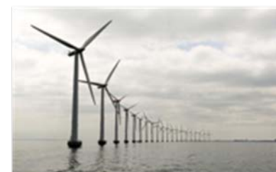
Offshore Power Generation
