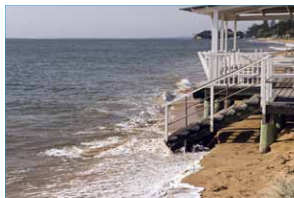
Erosion caused by rising sea levels due to global warming.
