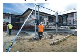
A high-lift hydraulic jack, developed by local firm Smith Cranes and Construction, provides an innovative solution to repairing earthquake damage to customers' homes in New Zealand. IAG was the first insurer to use this system. The home pictured was lifted and held at 2.7 metres for three weeks while the damaged concrete foundation pad was broken up, removed and replaced with a new foundation.
