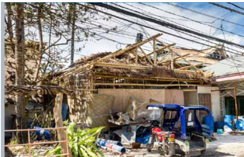
Boracay, Philippines, November 2013: building lies in ruins following Super Typhoon Haiyan.
